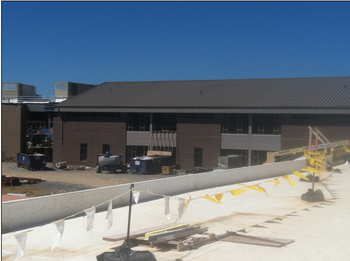
Figure 2: Standing Seam Metal Roof (Property of Mascaro Construction)
