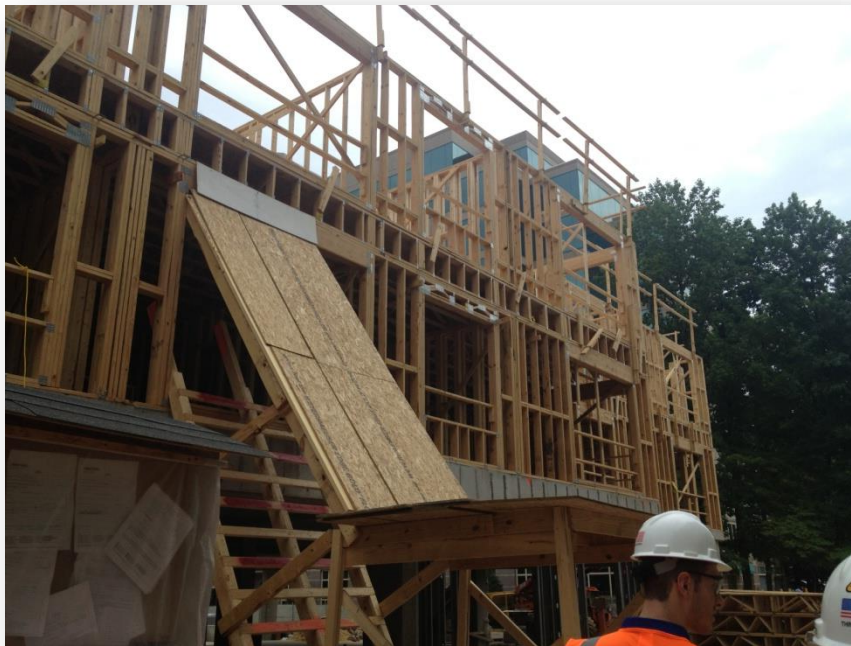
Figure 18: A personally taken picture of the early stages of a stick-built multi-family housing project.
