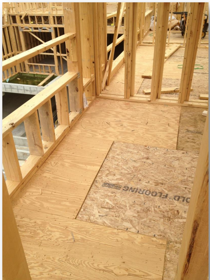
Figure 19: A picture taken at a stick-built multi-family residential building. Notice the higher resistant wood along the exterior wall.
