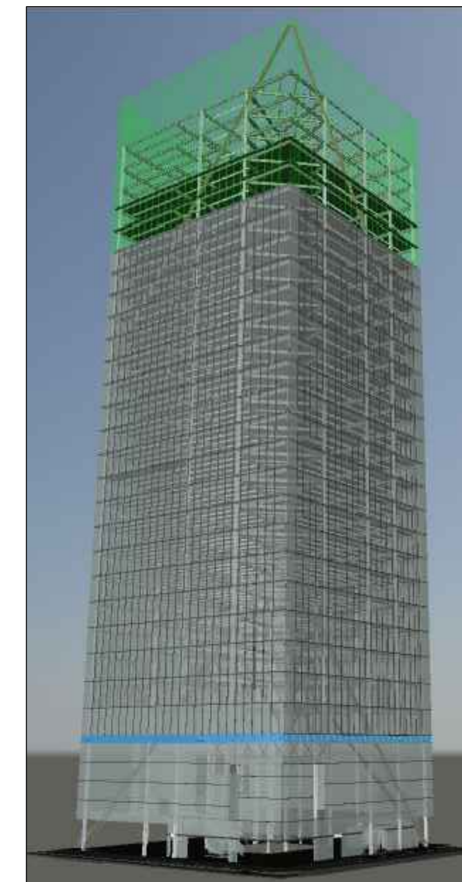
April 30, 2014: Final series of external lateral bracing has been installed. Facade rapidly catches up to sequencing plan to complete exterior the building. Following decking installation, roof work will commence. MEP work moves into the upper levels of 350 Mission.
