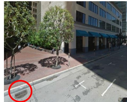
Appendix Figure 17: A storm water drain on Fremont street was chosen to discharge groundwater after being removed from the excavation site.
