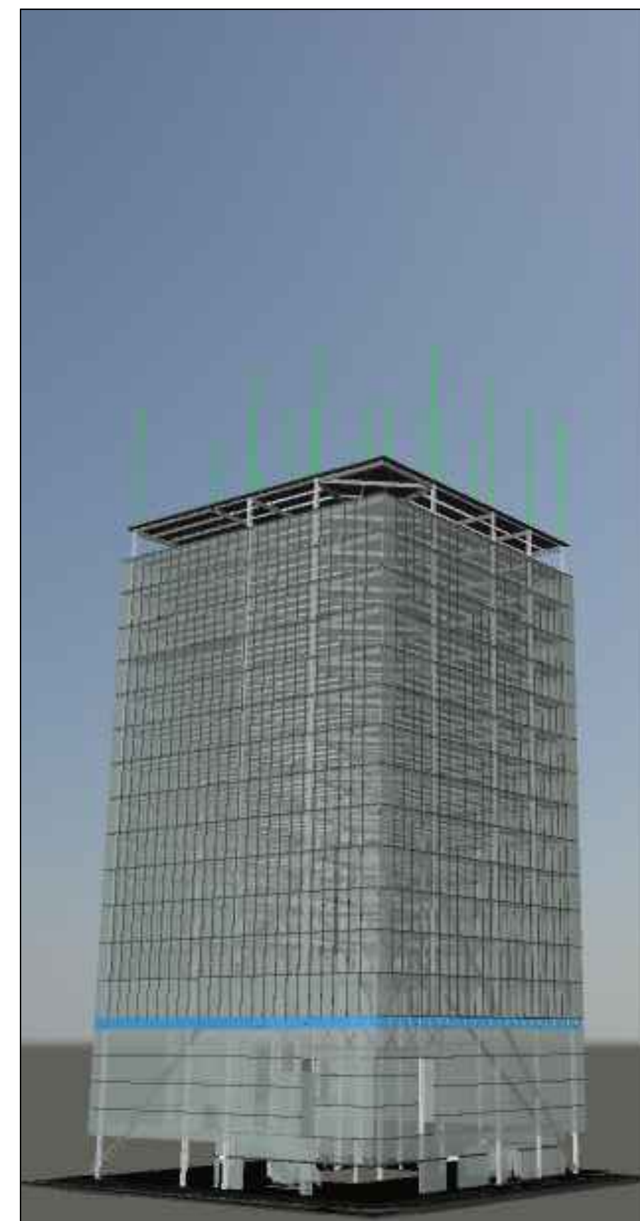
January 30, 2014: Structural work begins on floors 17-20. Facade lags slightly to prepare for installation of next level of exterior lateral beams.
