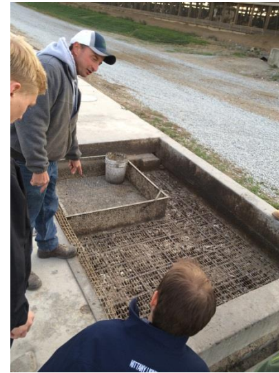
Above: the team investigates a grate used to filter waste materials from grease. The farm uses waste grease from local businesses to produce methane.
