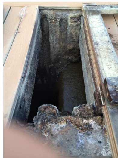
Digested products leaving the digester. The leftover materials are used to make bedding for animals at the farm.
