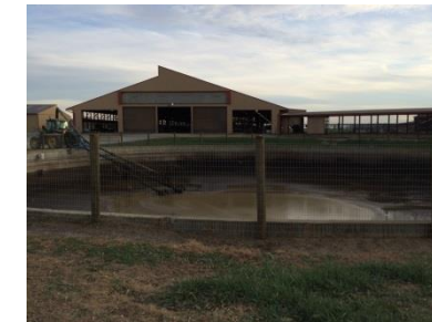
Filtered excess materials from the digester were stored in a pool.
