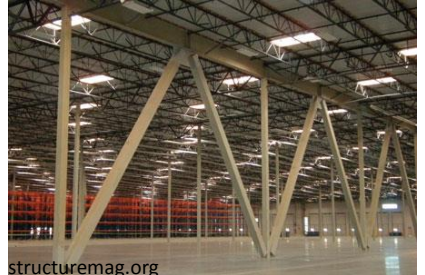
Concentric/Eccentric Brace
