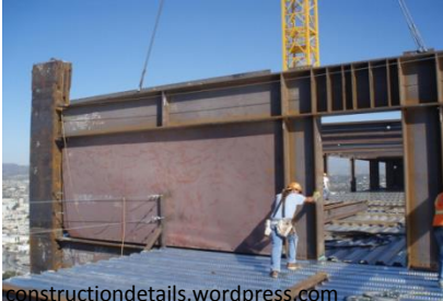
Steel Plate Shear Walls
