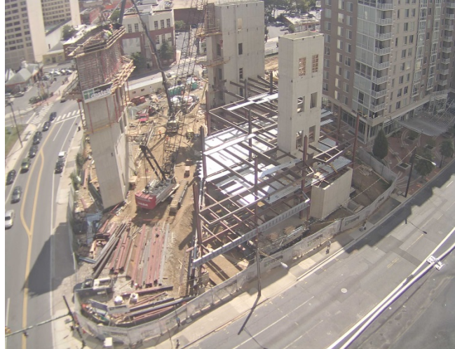
Figure 7 Superstructure Crane Placement (Provided by Multivista.com)
