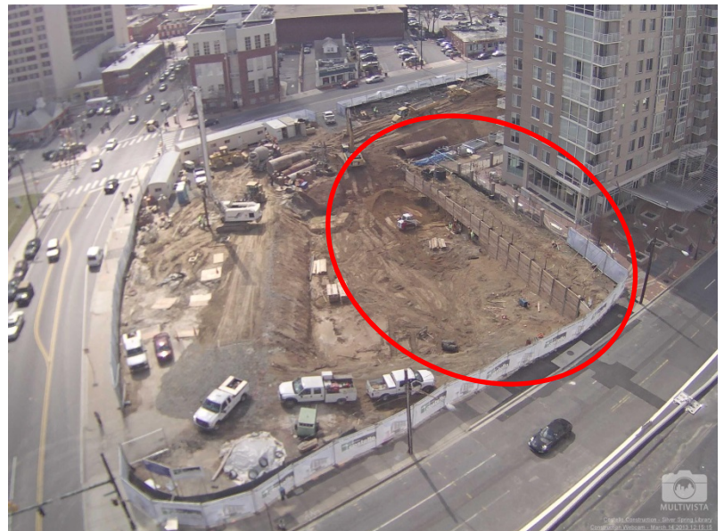
Figure 1 Excavation & Lagging (Provided by Multivista.com)
