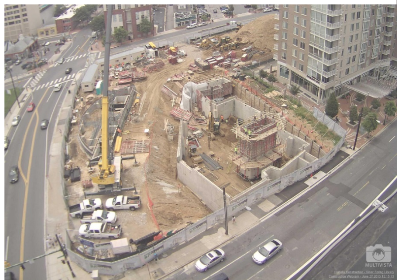
Figure 2 Foundation Walls & Shear Walls Installation (Provided by Multivista.com)
