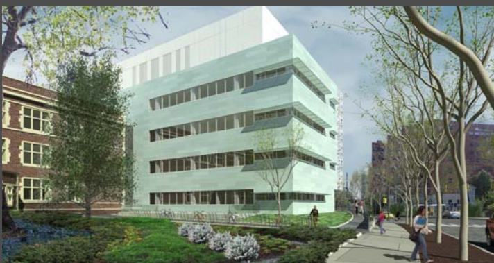
Looking South-East at copper clad block facade
