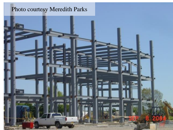
Figure 6: Photograph during erection of HSS framing
