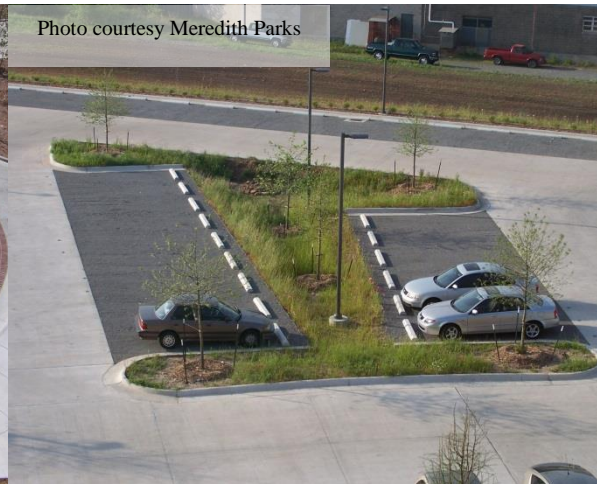
Figure 87: Porous pavement used in parking areas
