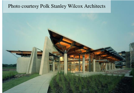
Figure 100: Exterior view of interior artificial light
