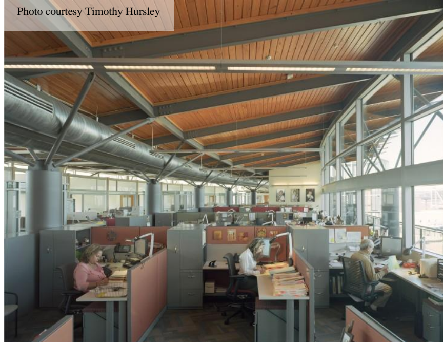
Figure 97: Natural daylighting in interior of building
