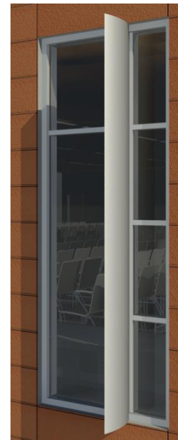
Figure 20. Façade complemented by glazing
