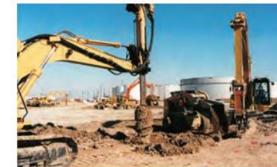
Houston Fuel Oil Terminal Company Houston, Texas
