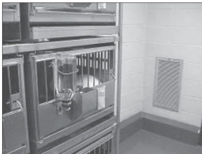
Figure 3. Exhaust air grille located near floor in an animal housing room.
