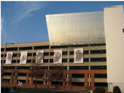
The façade of the parking structure consists of reinforced concrete and brick. Like typical parking garages, many openings in the façade are needed to ventilate the area from car exhaust. This means that the building envelope of this part of the building does not give any protection from the elements.
