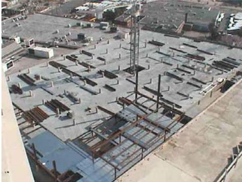
Sigal Construction Corporation was the project manager for the Iceplex. They acted as under a design-bid-build delivery method. The staging area for the new 8th and 9th levels was located on the 7th level of the existing parking garage.
