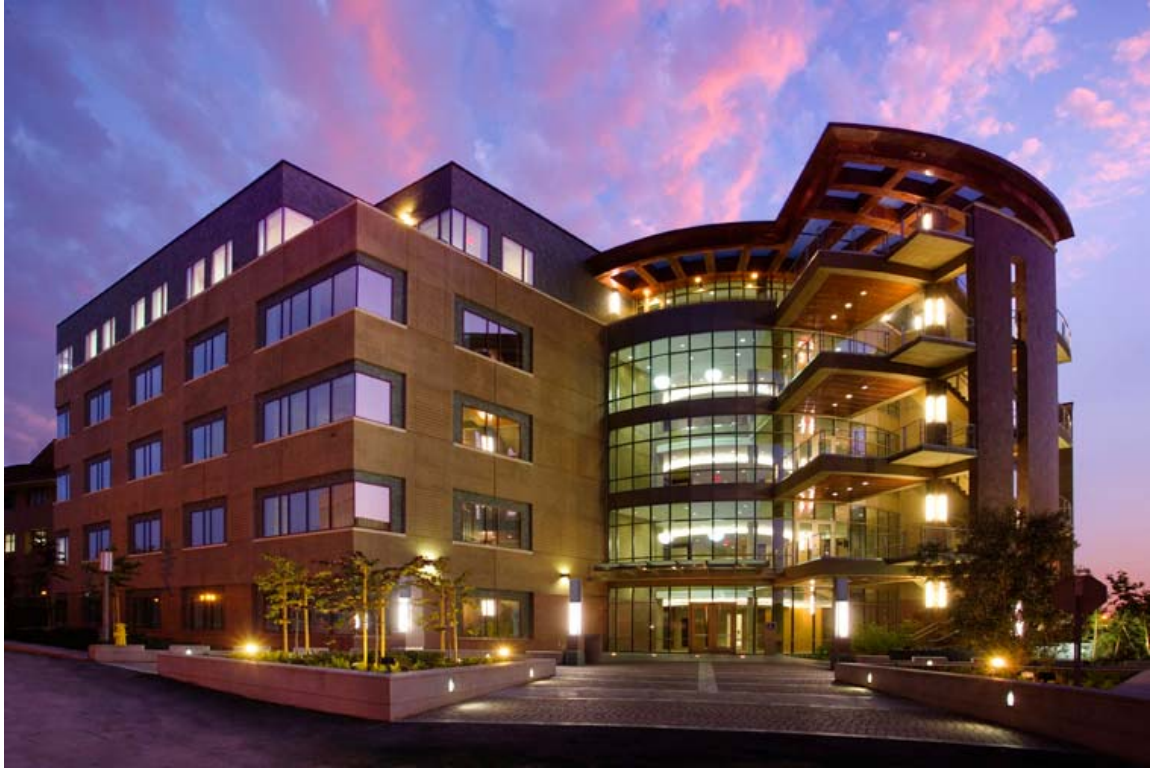
Plaza & Façade at Night
