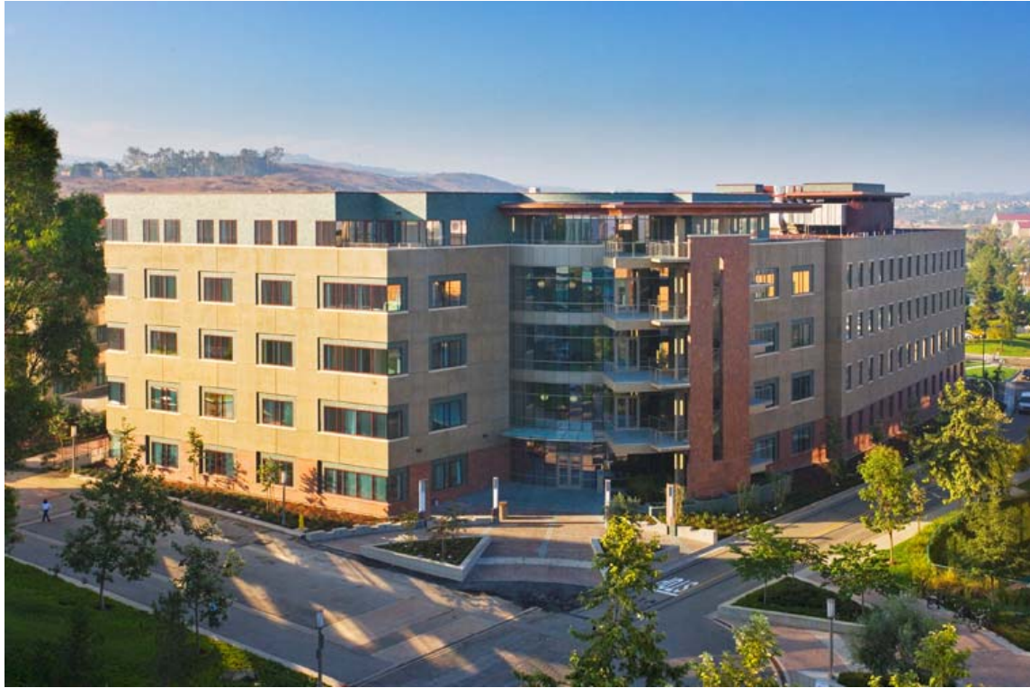
Plaza & Building Façade
