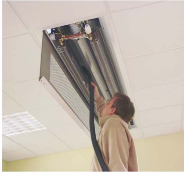
Figure 18: Maintenance Personnel Cleaning a Chilled Beam
