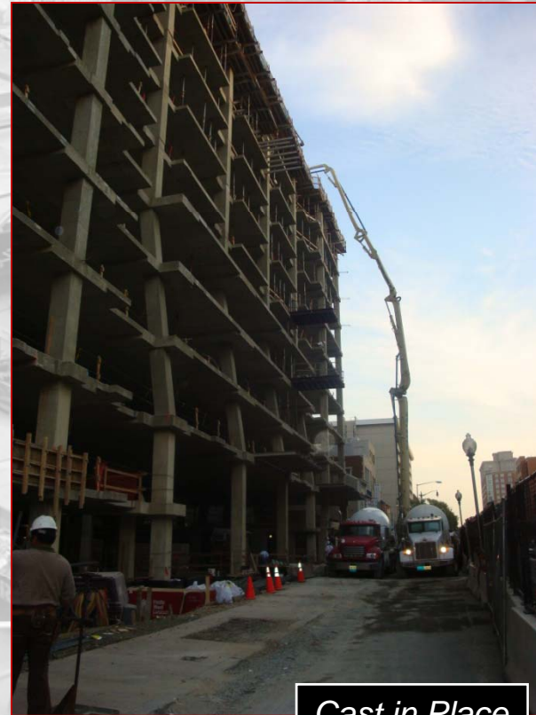
Cast in Place
