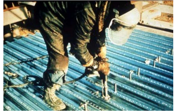
Fig10. Installation of Shear Studs
