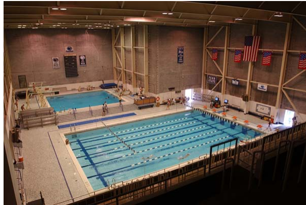
Figure1-1: Natatorium with steel structural system. Courtesy of Penn State
