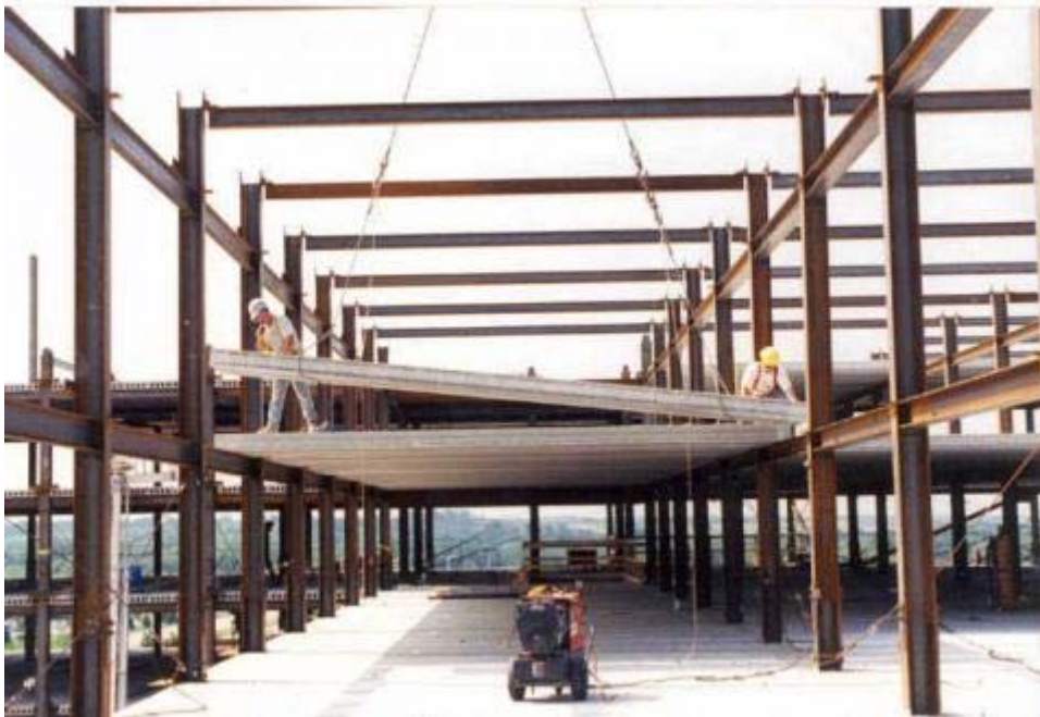
Figure 11 – A precast hollow core slab on steel beams during construction
