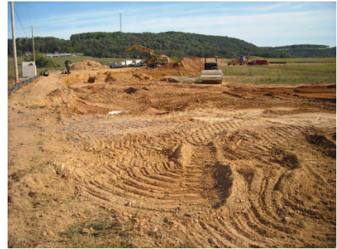
Figure 7: Beginning of excavation phase
