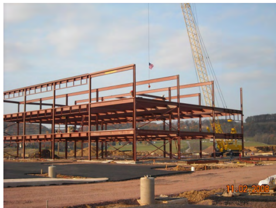
Figure 9: Steel frame construction
