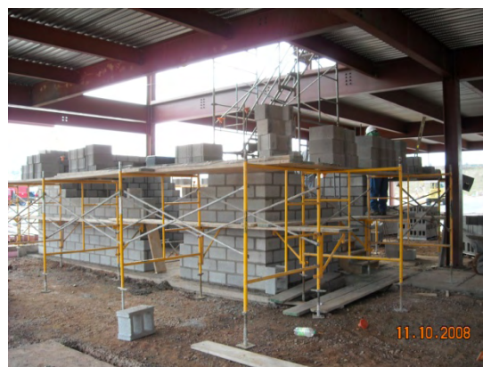
Figure 4: Elevator shaft 12" CMU walls
