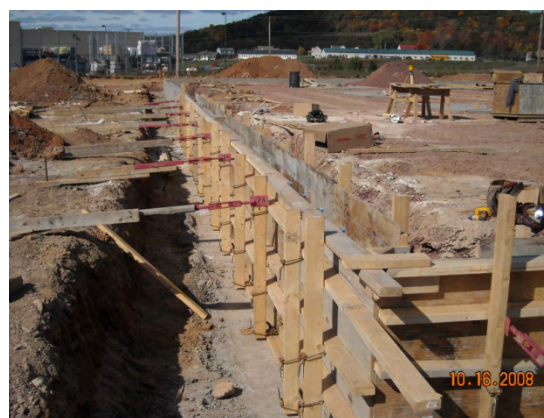
Figure 2: Concrete foundation formwork
