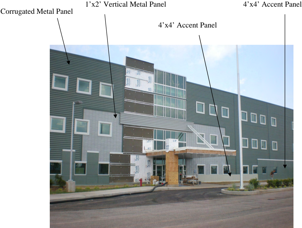
Figure 5: Various metal panels in curtain wall system
