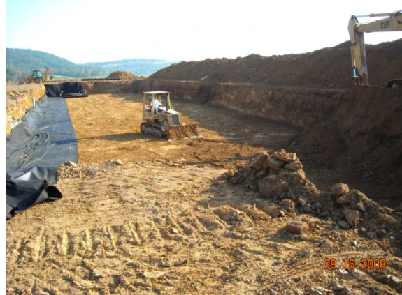
Figure 11: Excavation of foundations
