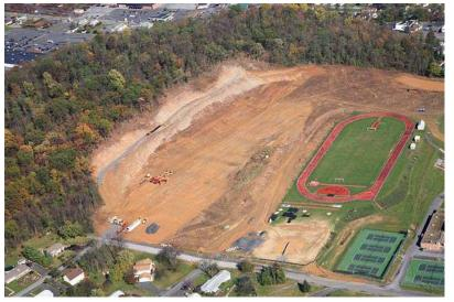
Excavation efforts critically drive early phases of the construction process. The site is located on a ridge north of the current school. Shown in the figure, extensive excavation and site work need to be completed before building construction can begin. Site work for this project also includes the drilling of wells for the geothermal mechanical system. The location of the site also calls for a long retaining wall along the north edge or rear of the site. The construction
