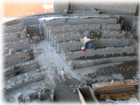
Figure 2: Installation of lecture hall structure
