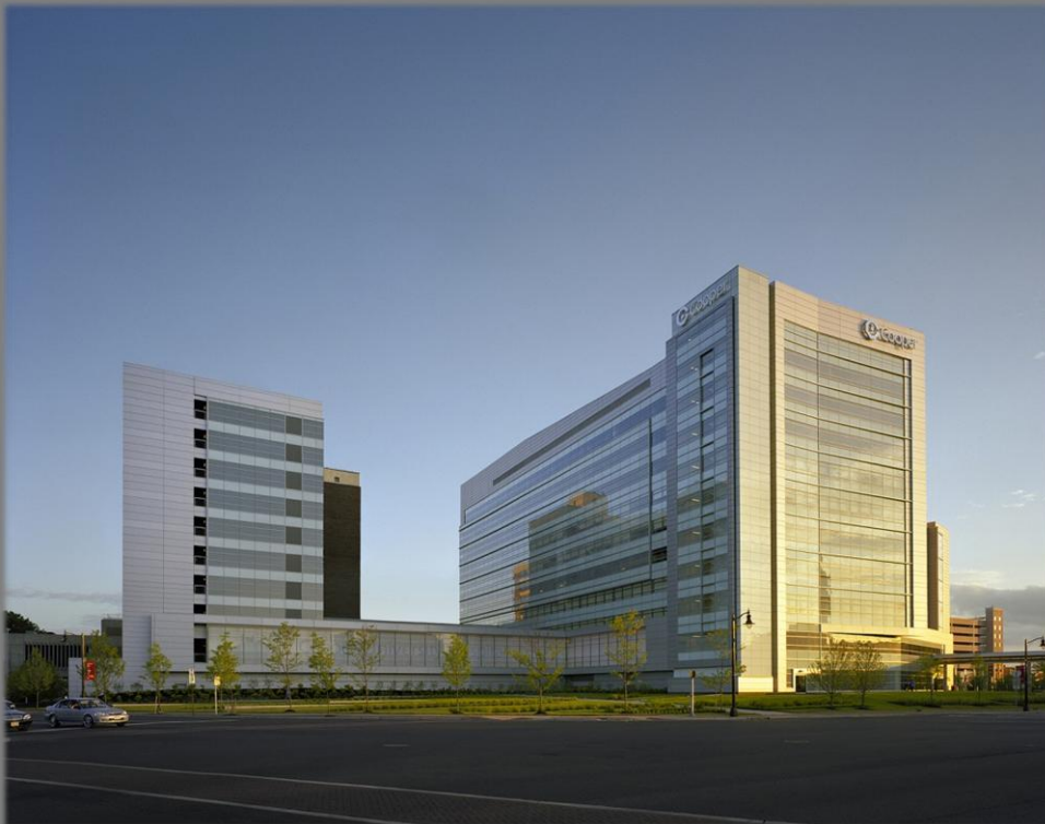
Roberts Pavilion Camden, NJ
