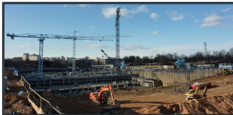
Figure 1: Construction of the Reston Station Garage
