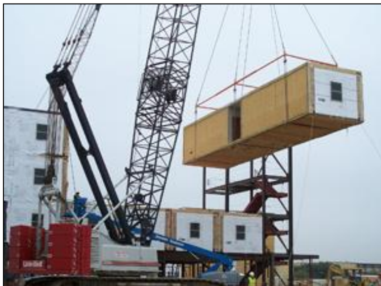
Figure 2 Example of Crane Setting Modular Units Picture Courtesy of TexasConstruction.com
