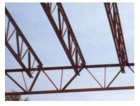
• Figure 16 – Open Web Joist Example
