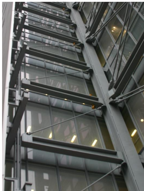
Figure 10: Cantilevered bays from exterior
