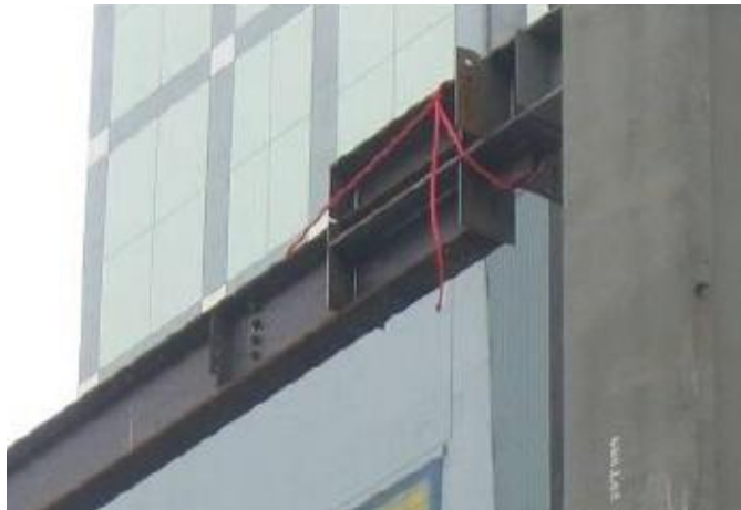
Figure 8: 'Dog-leg' beam prior to metal deck installation, courtesy of Thornton Tomasetti
