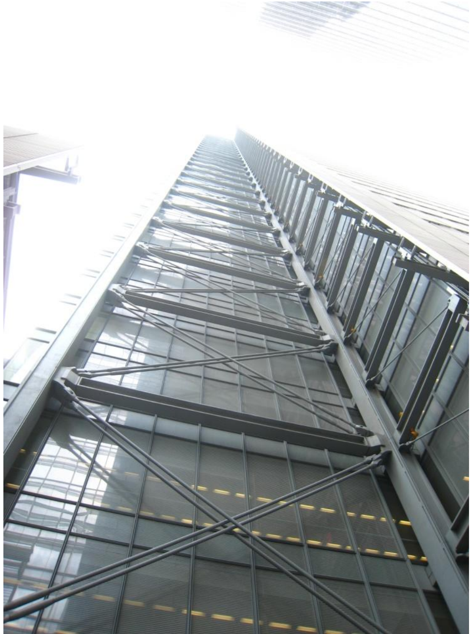
Figure 127: Exterior X-bracing
