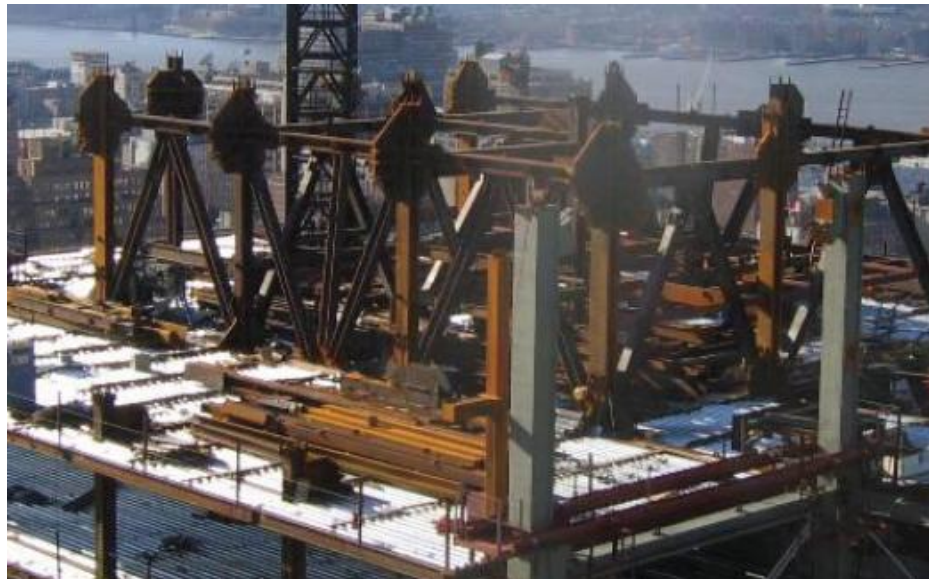
Figure 135: Core bracing during construction, courtesy of Thornton Tomasetti
