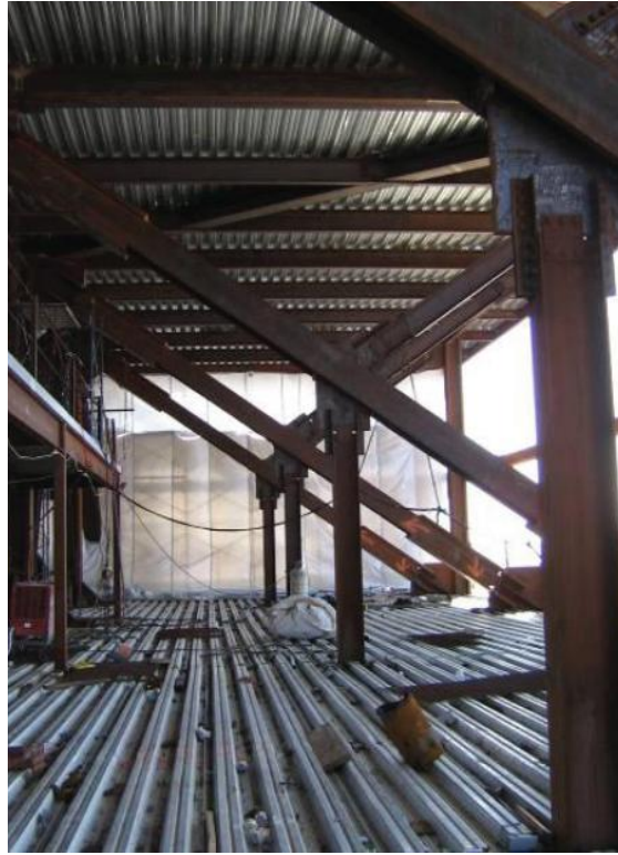
Figure 134: Outrigger bracing on mechanical floor, courtesy of Thornton Tomasetti
