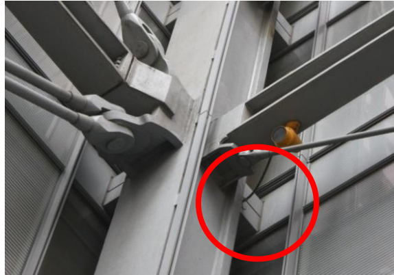
Figure 9: 'Dog-leg' penetrating building envelope
