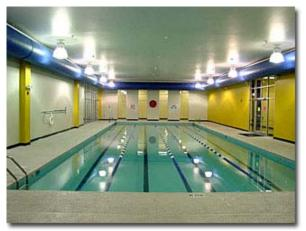
Figure 5-3: Duct Sox applied in a natatorium. Courtesy of Duct Sox
