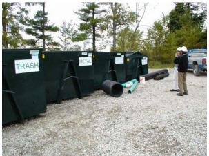
Figure 6-2: Construction waste recycling area. Courtesy of the State of Vermont.
