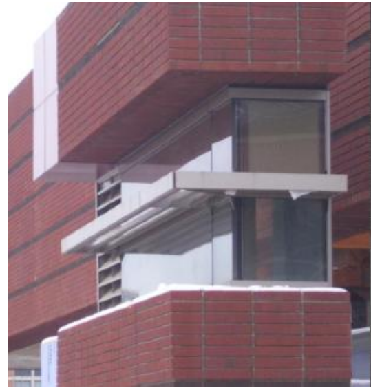
Figure 2: Mockup of building enclosure, including pre-cast panels courtesy of Ryan Solnoksy
