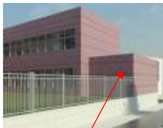
Figure 4 —Cooling Tower Hidden from outside
