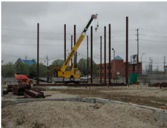
Steel Erection by Mobile Crane
