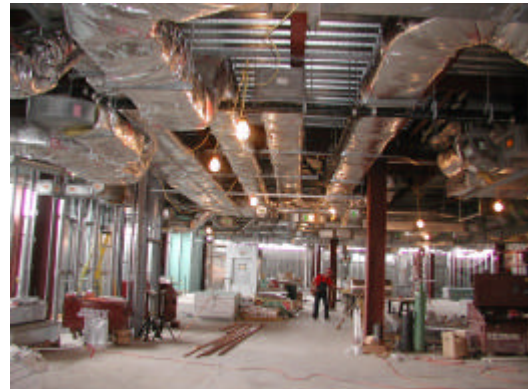
Sheet Metal Ductwork Installation
