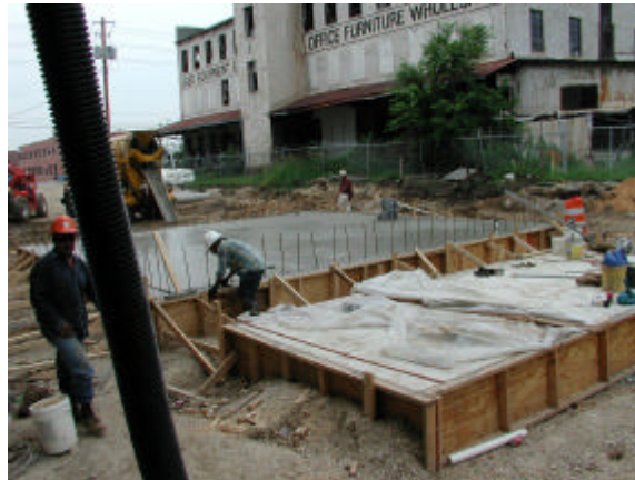
Typical Plywood Forming and Bracing
