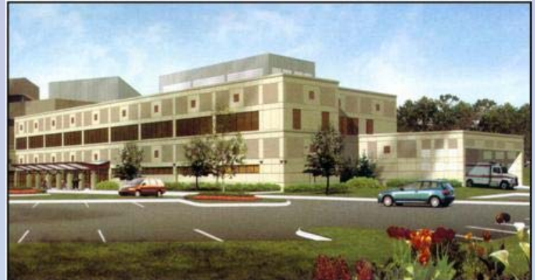
Courtesy of Leach Wallace Associates
