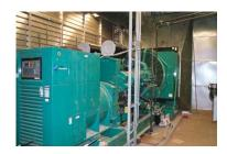
power from a 1250kW/1562kVA Diesel Generator to keep life support systems functioning at all times. Multiple surge suppression devices are located on each major panel to ensure safety of the system from overload.
