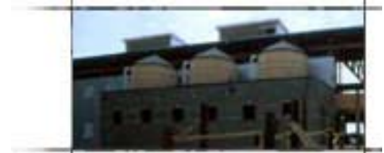
Figure 19: SWR Tanks @ CBFPMEC
