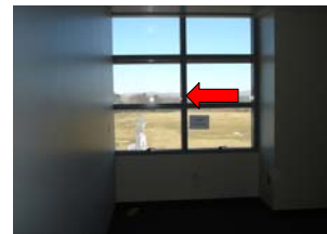
4 th Floor North Wall
