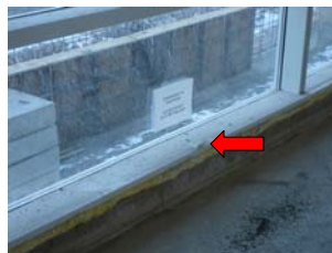
Sensor on Atrium Windowsill
