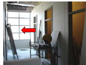
1 st Floor NW Corner
