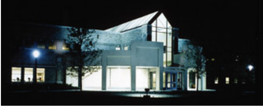
Fig.4 Kalwall emitting light at night
