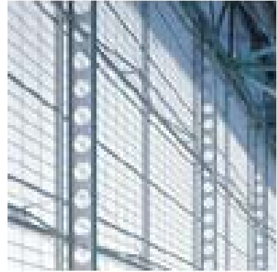
Fig.5 Light transmitting wall system
