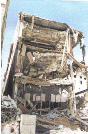
Figure 6: Restaurant Next to the Alfred P. Murrah Building
