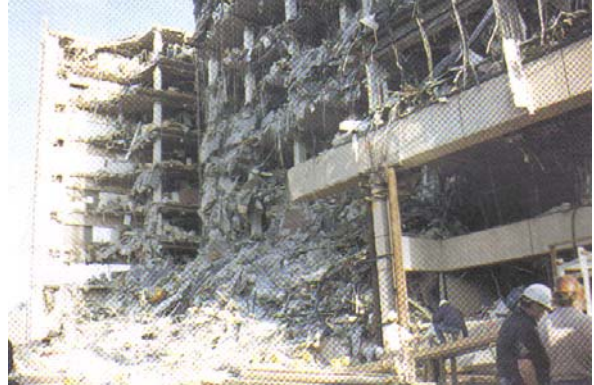
Figure 4: Damage to the North Side of the Alfred P. Murrah Building
