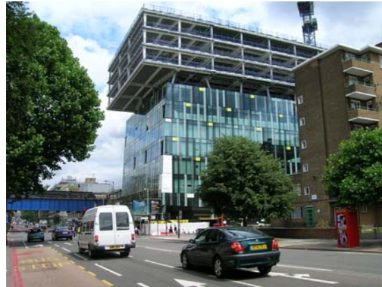
Figure 5.1 Palestra Under Construction
