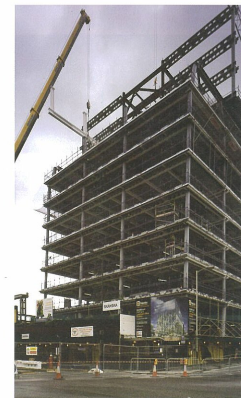
Lifting in the 9m cantilevers required a partial road closure.
