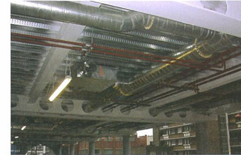
Enlarged holes in the web made service installation easier.
