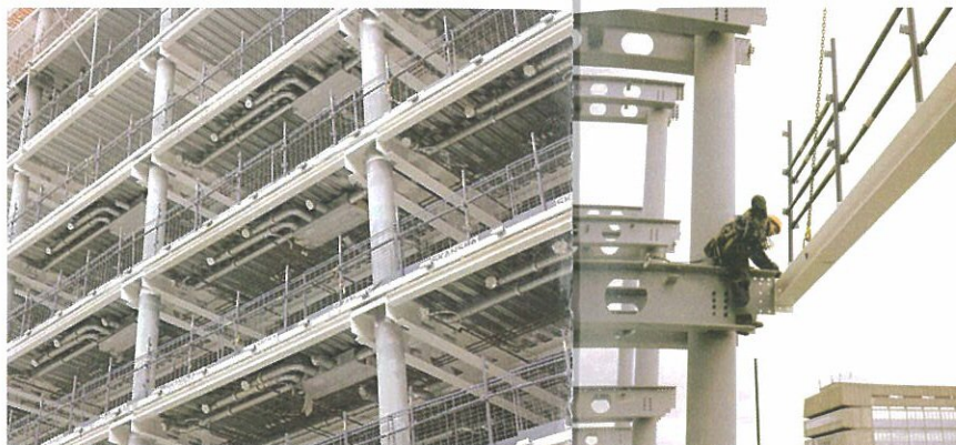
Installing the steelwork for the cantilever over Blackfriars Road
