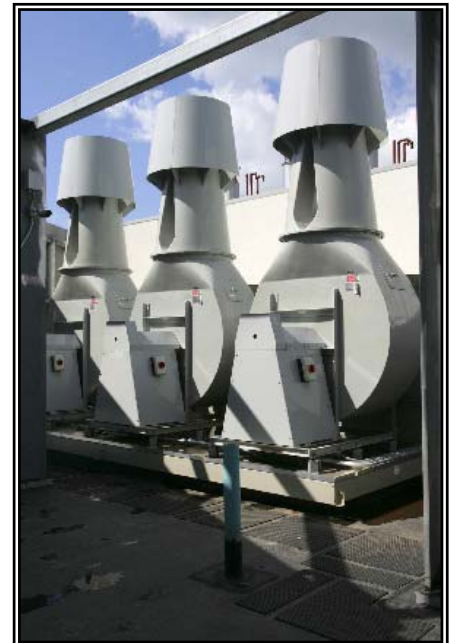
Figure XII: Laboratory Exhaust Fans
