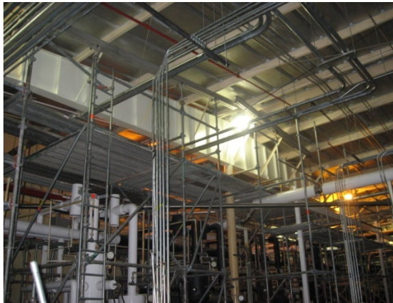
Image 5: Shows the original structural frame with repairs to return it to initial strength. Also shown is all of the processing equipment around it.
