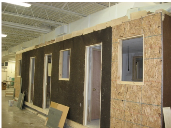
Image B.5: Hands on construction, interior finishing.
