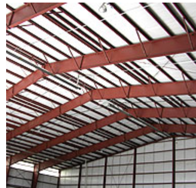
Image 3: Shows the structural system of a pre-engineered metal building. The frames are the larger beams that run the width, while the purlins are the smaller beams closer to the ceiling.
