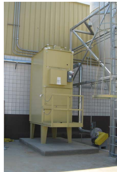
Image 7: Shows the exterior Make-up air units by AbsoluteAire that were used on Project Stallone.
