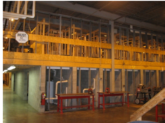
Image B.10: Hands-on plumbing class with water heaters on bottom and units on top.
