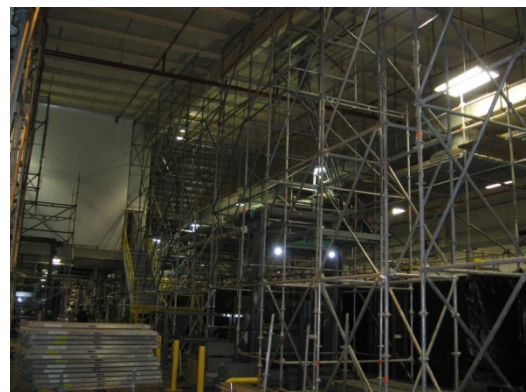
Image 4: Shows the extensive temporary bracing (Scaffolding) that was put in place to ensure the safety during unloading and repairs.
