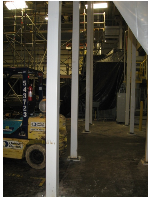
Image 6: Shows the newly installed stands, used to remove equipment load existing frames.
