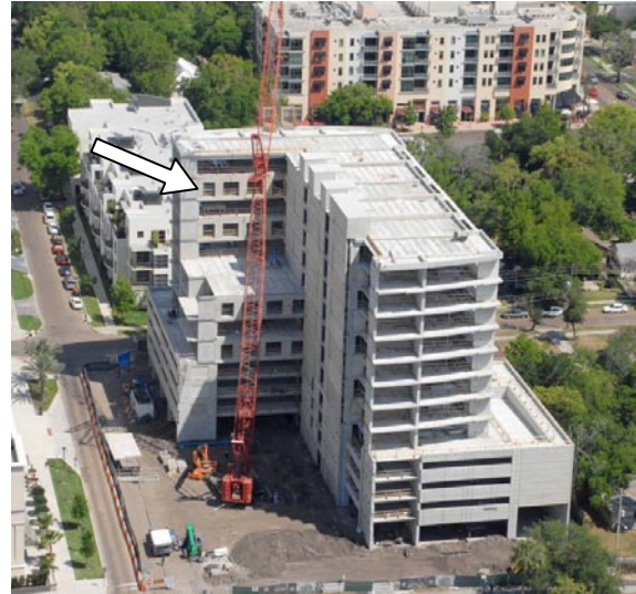
101 Eola Under Erection: Courtesy of Finrock Industries
