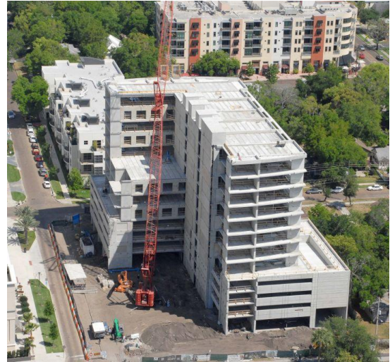
101 Eola Under Construction: Courtesy of Finrock Industries
