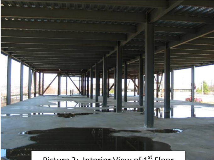
Picture 3: Interior View of 1 st Floor
