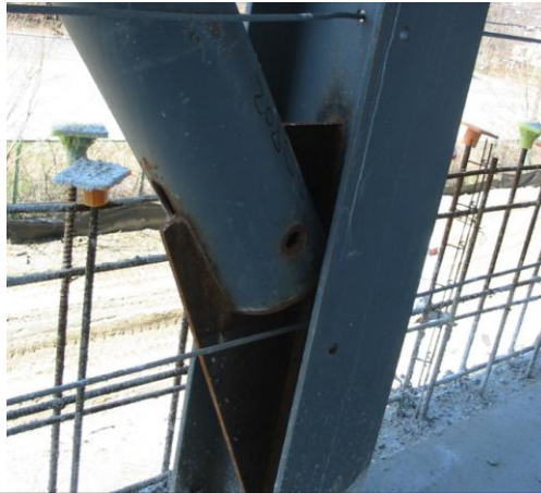
Picture 4: Typical Lateral Brace Connection
