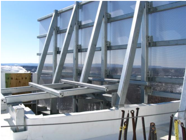
Picture 6: Penthouse Mechanical Screen
