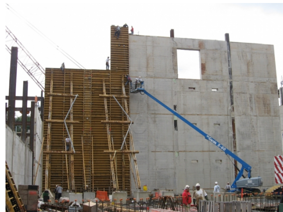
Figure 2.5: Pouring of concrete shear wall
