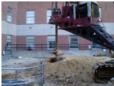
Caisson Being Drilled
