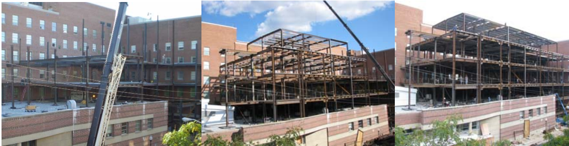
Structural Steel Progress Photos: 9/5/08, 9/15/08, 9/23/08
