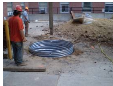
Caisson Excavation support
