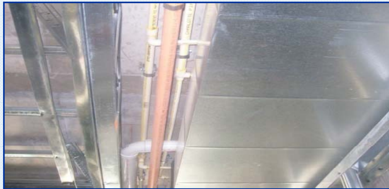
CPVC piping in ceiling space
