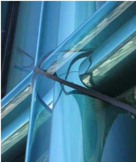
Figure 14 – Typical Mullion Intersection
