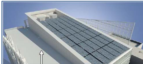
Figure 4: Solar Panels on tower roof
