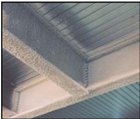
Figure 21: Example of spray on fireproofing applied to beams and girders.
