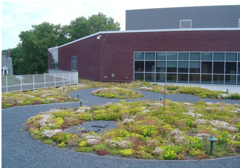
Figure 24 – Milton Hershey School Health Center (courtesy of American Hydrotech, Inc.)
